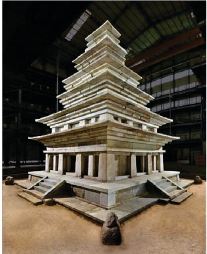
In June 2018, the Cultural Heritage Administration unveiled the famous stone pagoda at Mireuksa Temple in Iksan, National Treasure No. 11, after 20 years of repair and restoration.
